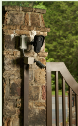
Electric & Existing Structure / Pole
