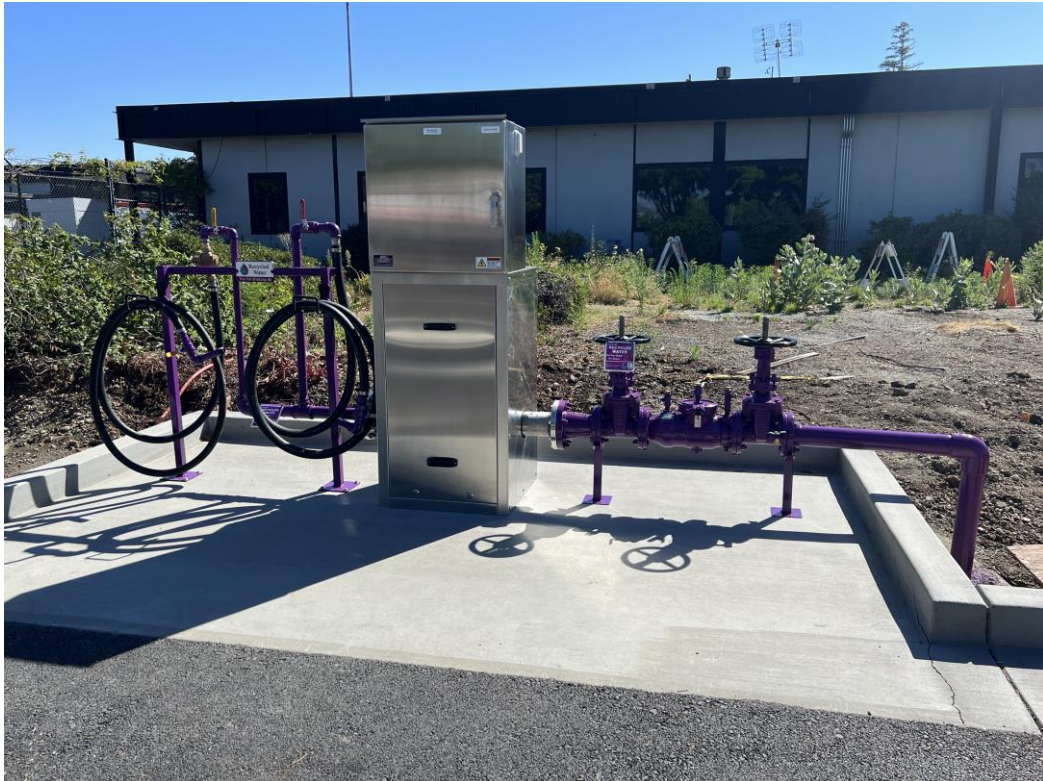
Automated Residential Recycled Water Fill Station
