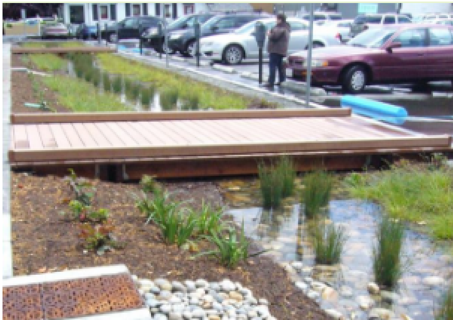
Bio-retention Area Example – San Mateo County Water Pollution Prevention Program
